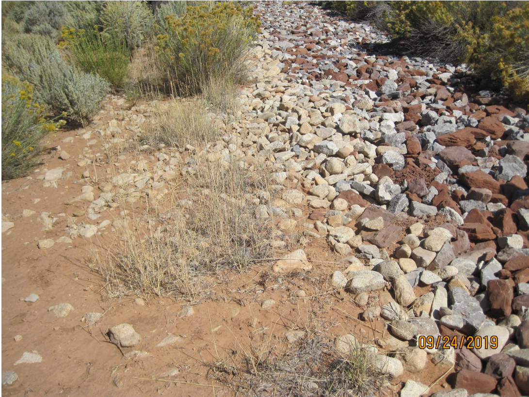
Figure No. 5, Sediment transport into toe apron, east side slope
