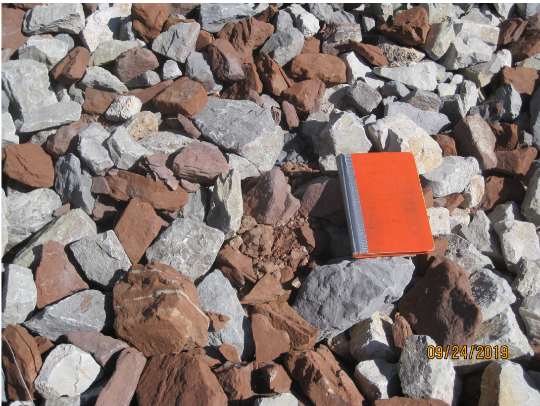
Figure No. 6, Break down of sandstone rock, east side slope apron
