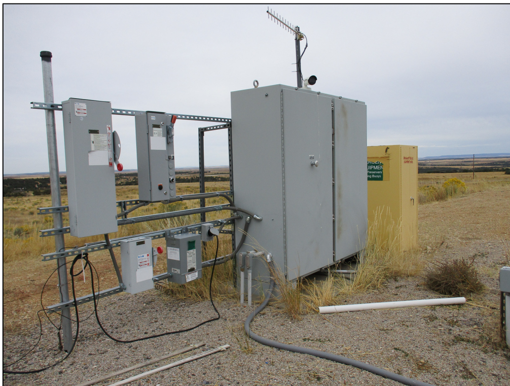
PL-16. Pond 4 LCRS/LDS Control Cabinet
