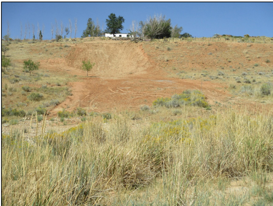
PL-28. Embankment on Property MP-100181 Showing Repaired Water Line Break Erosion
