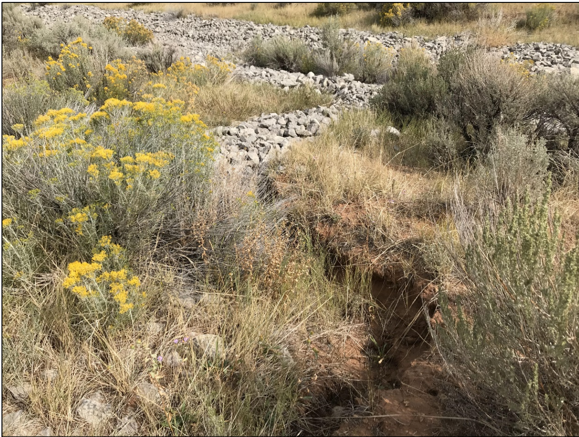
Figure B-2. West Drainage Channel Erosion
