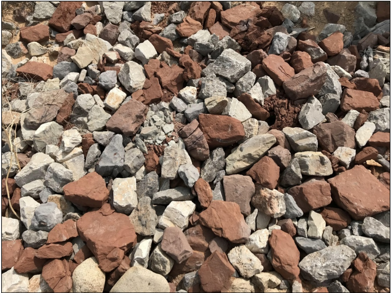
Figure B-6. Breakdown of Sandstone Rock, East Thickened Riprap Toe
