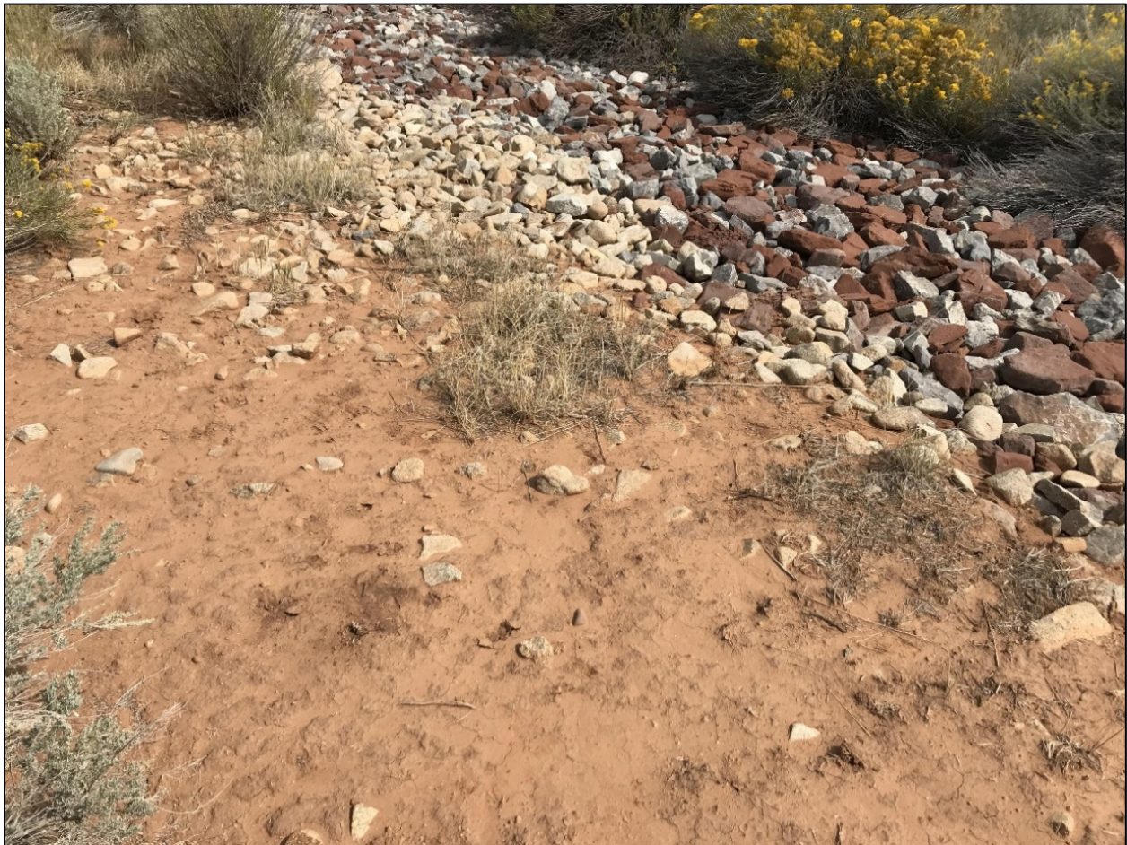
Figure B-5. Sediment Transport into East Thickened Riprap Toe
