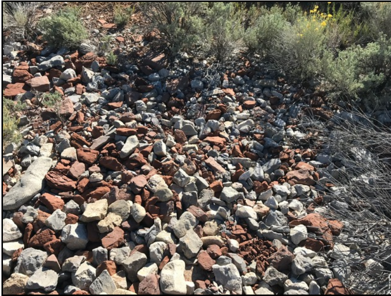
Figure B-7. Breakdown of Sandstone Rock, East Thickened Riprap Toe
