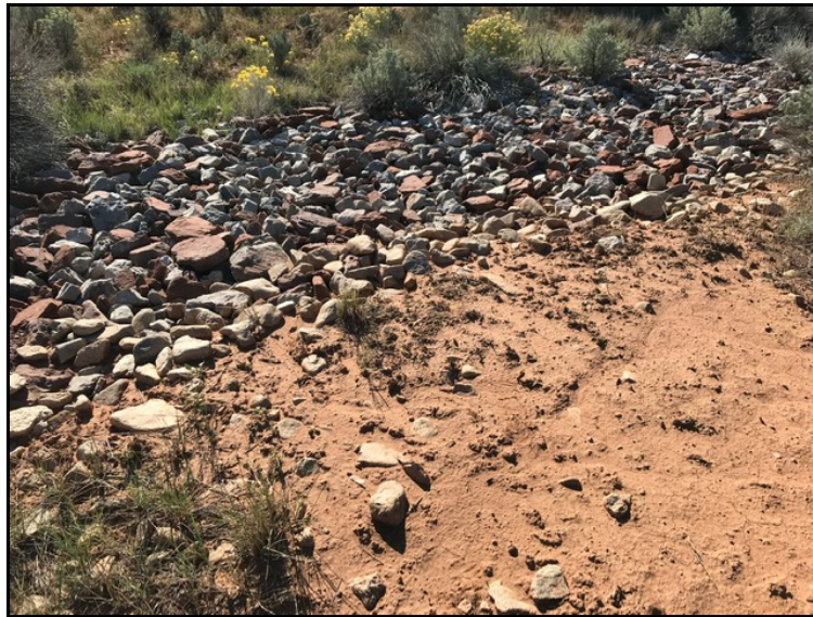
Figure B-5. Sediment Transport onto East Thickened Riprap Toe
