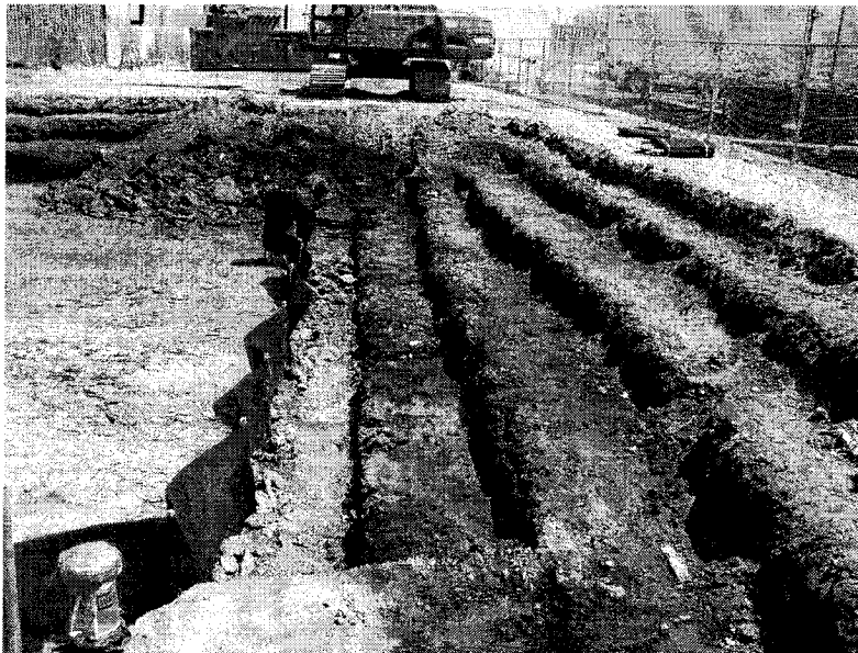
Fig. 2 - Dark lens of material in the excavation
