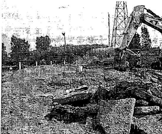
Engineering controls included water misting for dust suppression
