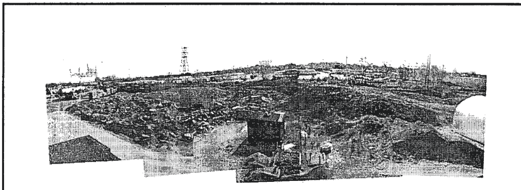
Configuration of Linde Site Spoils Pile - May 2005
