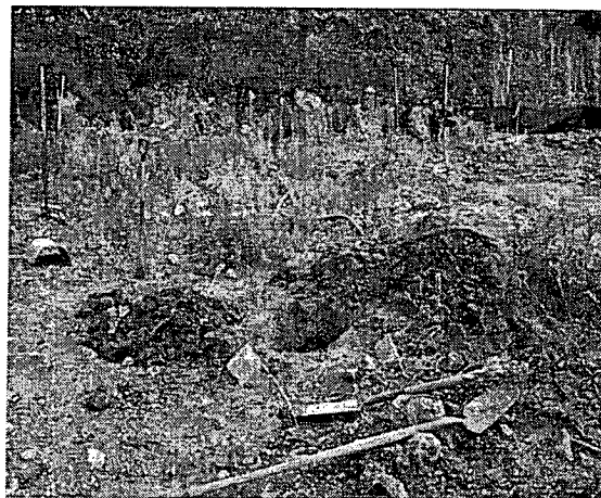
Hand digging was performed to verify the location of subsurface utilities
