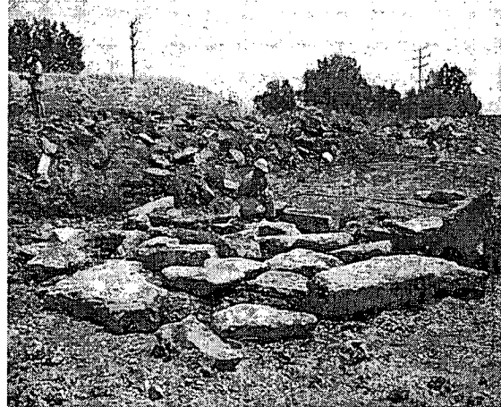
Concrete slabs were rinsed with water, laid flat to dry, and scanned for potential radiological contamination.
