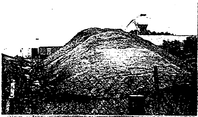
The spoil piles were recently sprayed with a gray polymer-type coating, which has stabilized them until their scheduled removal this fall.
