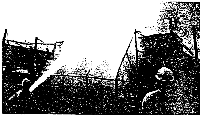
Engineering controls and measures, such as dust suppression and sediment traps, are utilized to limit migration of contaminants away from cleanup sites.
