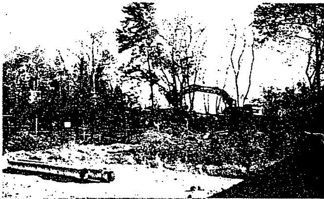
Crews begin clearing activities for the HISS railspur construction and sewerline encasement.
