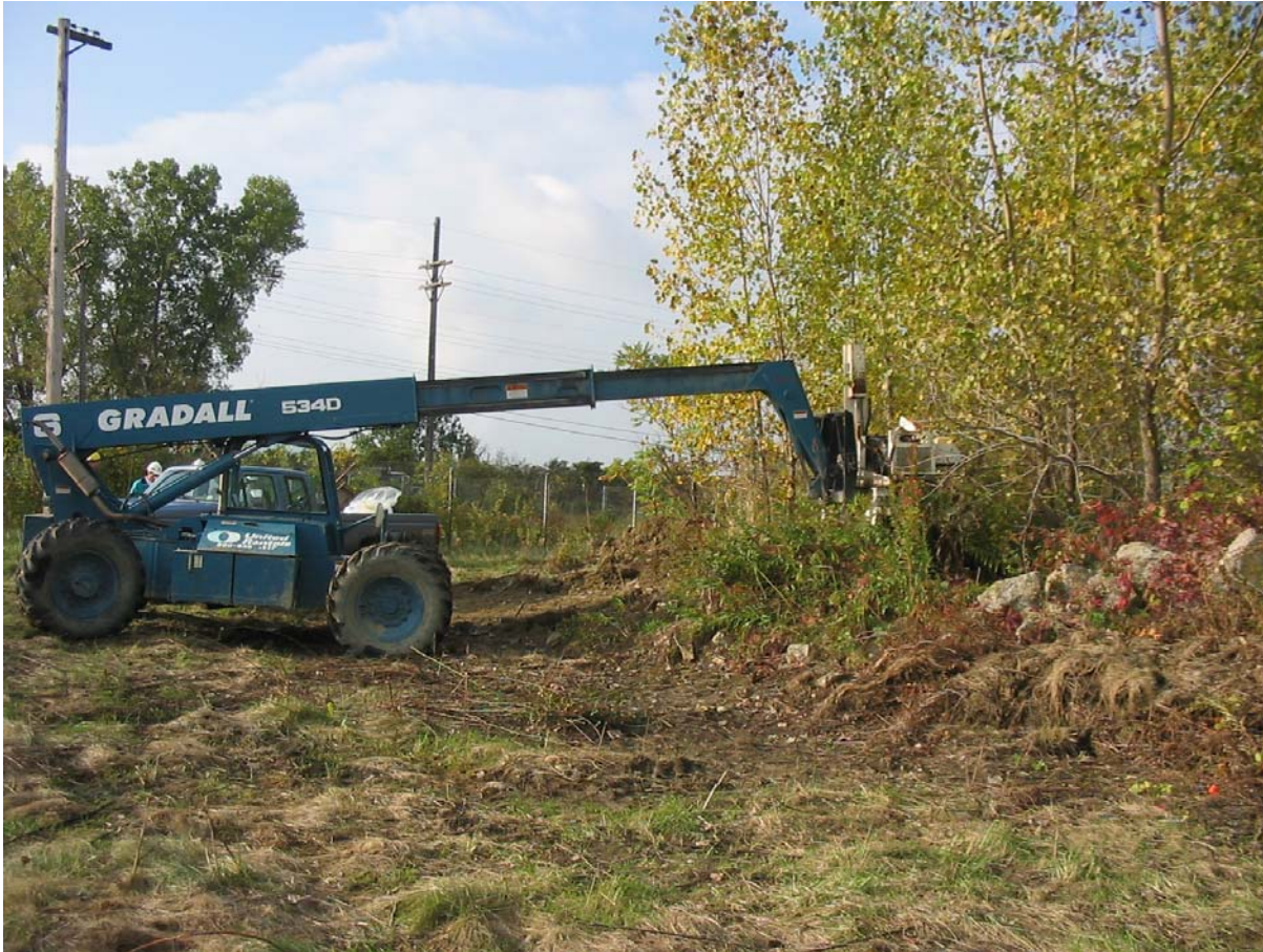
Figure 3-2. Skid-Mounted Earthprobe™ Rig Being Positioned on Rubble Pile at PVS070.
