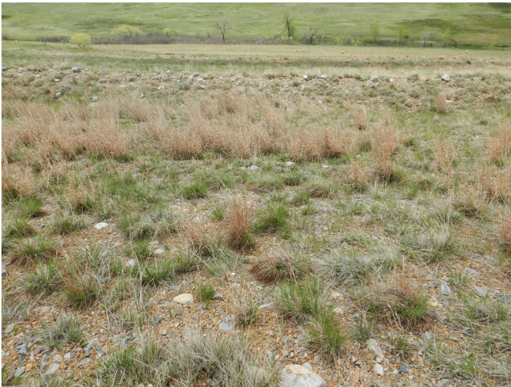
Figure 5. Looking South at Berms 4–7, Which Were in Good Condition
