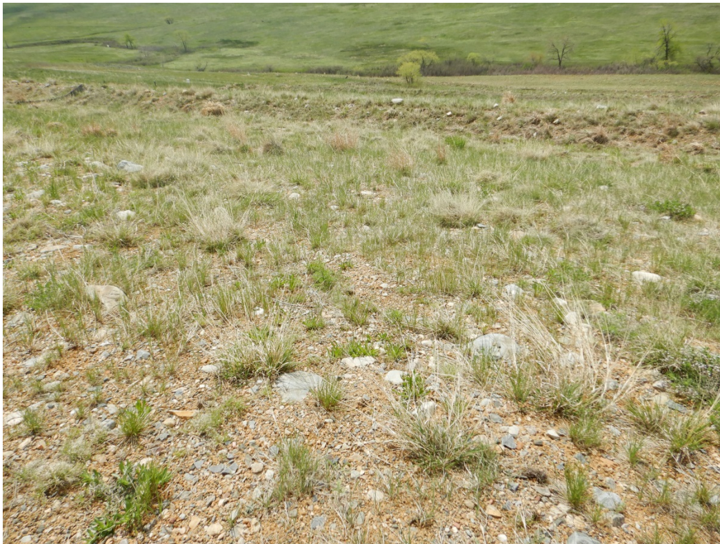
Figure 4. Looking Southeast at Berms 4–7, Which Were in Good Condition
