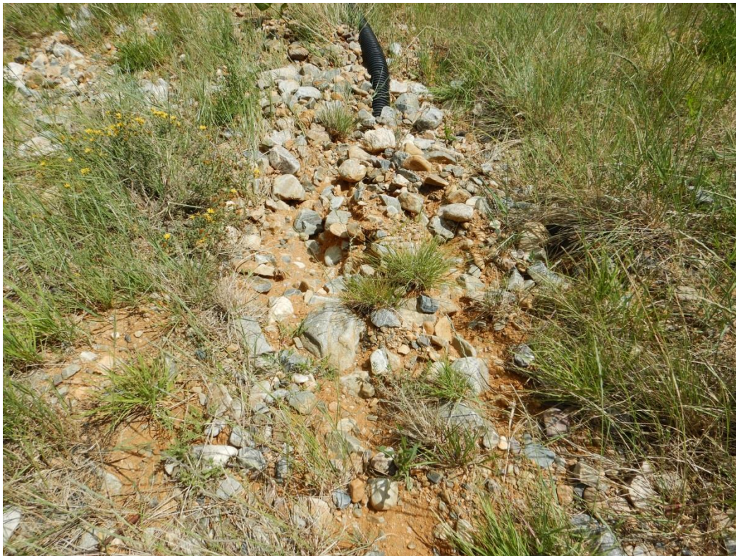
Figure 4. Looking Down at Erosion on East-Central Berm 5
