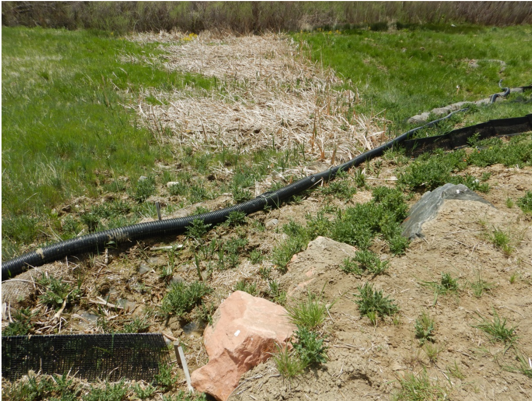
Figure 2. Looking South to the Toe of the Regraded 2017 Slump Area Blocking the Lower Segment of the EPC and the Well-Vegetated Area Where Surface Water is Currently Directed
