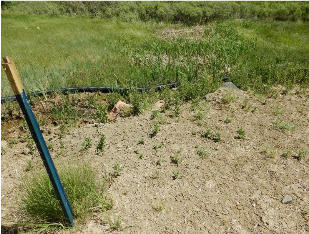
Figure 2. Looking South at the Toe of the Regraded 2017 Slump Area Blocking the Lower Segment of the EPC, and the Well-Vegetated Area Beyond Where Surface Water is Currently Directed
