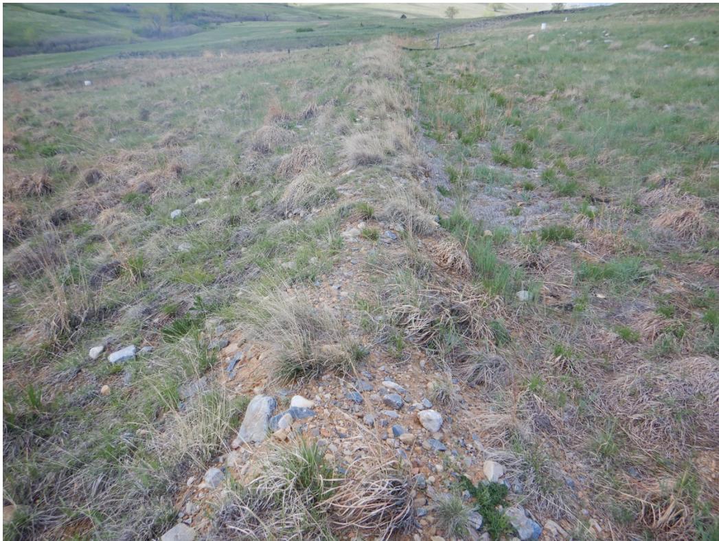
Figure 3. Looking West from the East End of Berm 2 to Berms 1–3, Which Were in Good Condition
