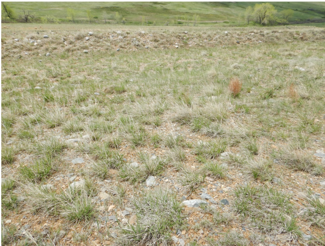
Figure 6. Looking Southwest at Berms 4–7, Which Were in Good Condition
