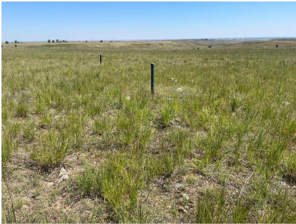
*Figure 5. Looking East-Northeast at the Top of the Landfill Cover, Which Was in Good Condition. Barometric gas vents for release of methane (left) and settlement survey markers (right) are strategically placed along the landfill's cover. No issues were found with barometric gas vents or settlement survey markers.*
