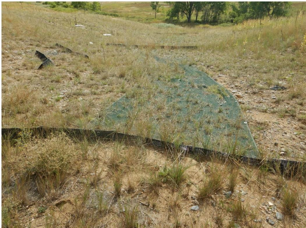
*Figure 5. Looking Southeast at the WPC, Where There Is Erosion Beneath the TRM and a Lack of Vegetation Along the Lower End of the WPC*
