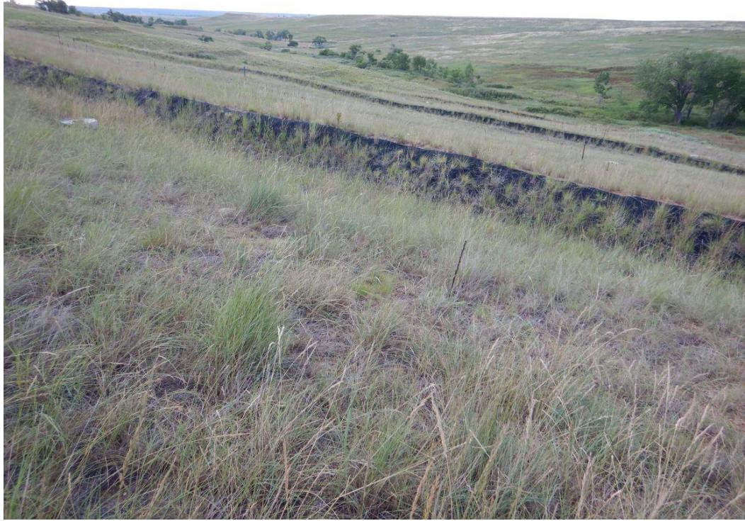
*Figure 2. Looking Southeast at Berms 1–3, Which Were in Good Condition*
