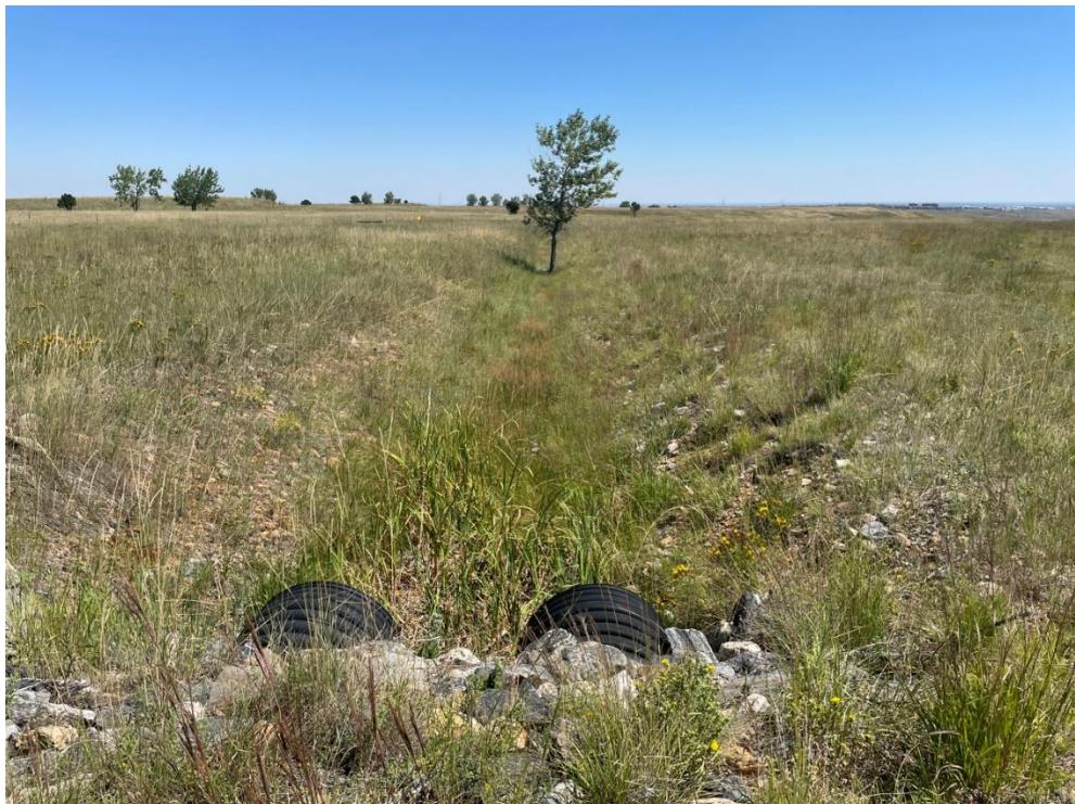
*Figure 2. Looking East-Northeast at the Northern Vegetation-Lined Perimeter Channel. This area has been designated as a wetland. All channels and culverts appear to be functioning properly.*
