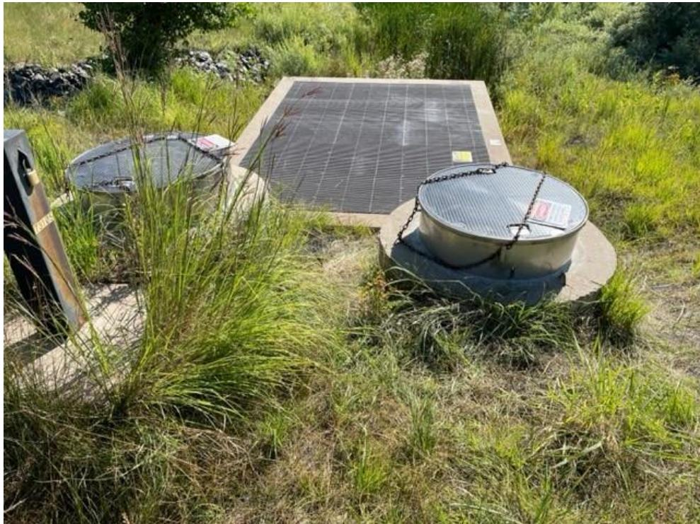
*Figure 1. Looking East at the Present Landfill Treatment System On 8/17/2023 After New Lids Were Installed, Which Will Be Safer and Easier to Operate. Small amounts of Bio-growth were removed from the North and South Manhole Outlet Pipes, treatment unit outlet pipe, and system outfall using a mechanical pipe cleaner as part of routine preventative maintenance. Bio-growth in the north manhole is scheduled to be addressed with the help of a subcontractor.*
