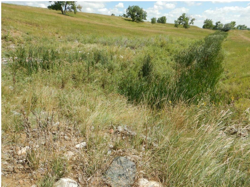
*Figure 9. Looking East-Northeast at the SID, Which Receives Groundwater from the ESSD Outfall and an Interceptor Drain on the Eastern Hillside and Had a Flow of 1–2 gpm*
