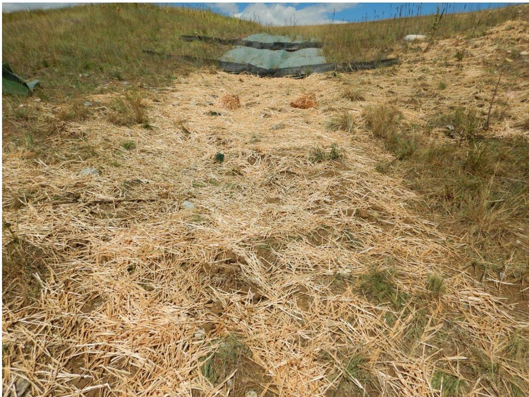
Figure 5. Looking West-Northwest at the WPC, Where Erosion Beneath the TRM and the Lack of Vegetation Along the Lower End of the WPC Is Being Addressed by Removing Sections of TRM With Little to No Vegetation, Laying Wood Straw, Reseeding, And Placing Erosion Controls Where Necessary.
