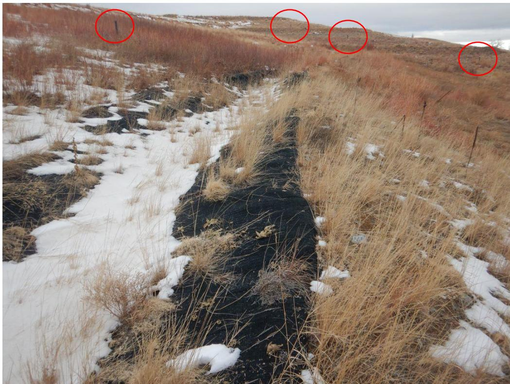
Figure 4. Looking East-Northeast at Settlement Monuments (Circled in Red) Strategically Positioned Along the Western Half of the Landfill, Which Were in Good Condition
