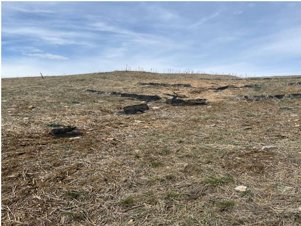
*Figure 5. Looking West-Northwest at the Lower End of the WPC, Where Three Rows of GeoRidges Had Signs of Being Trampled by Elk*
