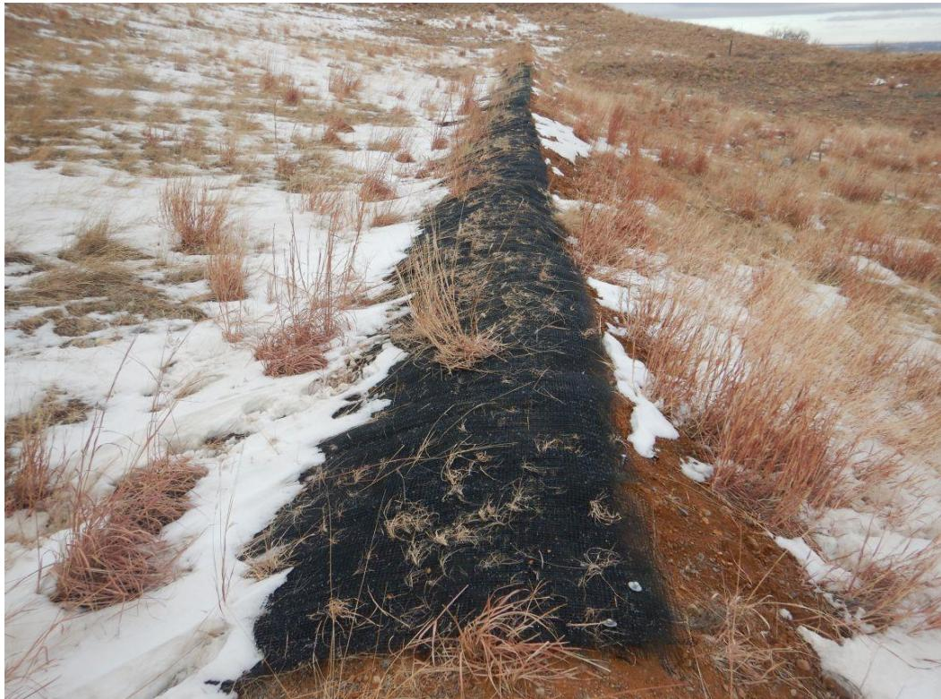
*Figure 3. Looking East-Northeast at the TRM on Berm 2, Which Has Remained in Good Condition Since Installation in December 2022*
