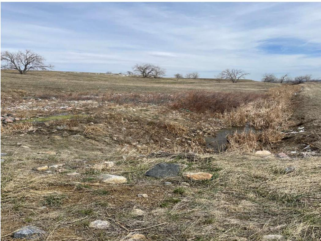
*Figure 10. Looking East-Northeast at the SID, Which Receives Groundwater from the ESSD Outfall and an Interceptor Drain on the Eastern Hillside and Had a Flow of 2–3 gpm*
