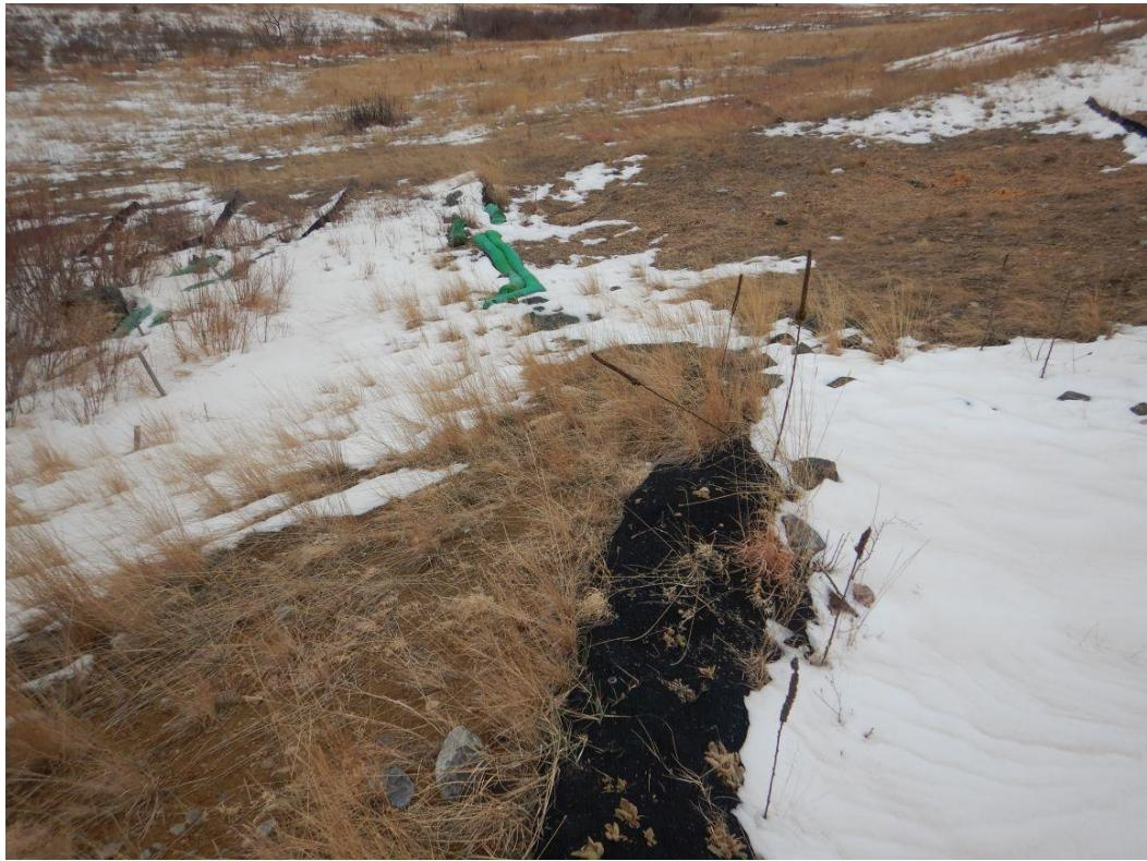
Figure 7. Looking West-Southwest at Wood Mulch Wattles Meant to Control Sediment at the Bottom of the WPC, Which Have Remained in Good Condition Since Replacement in August 2023
