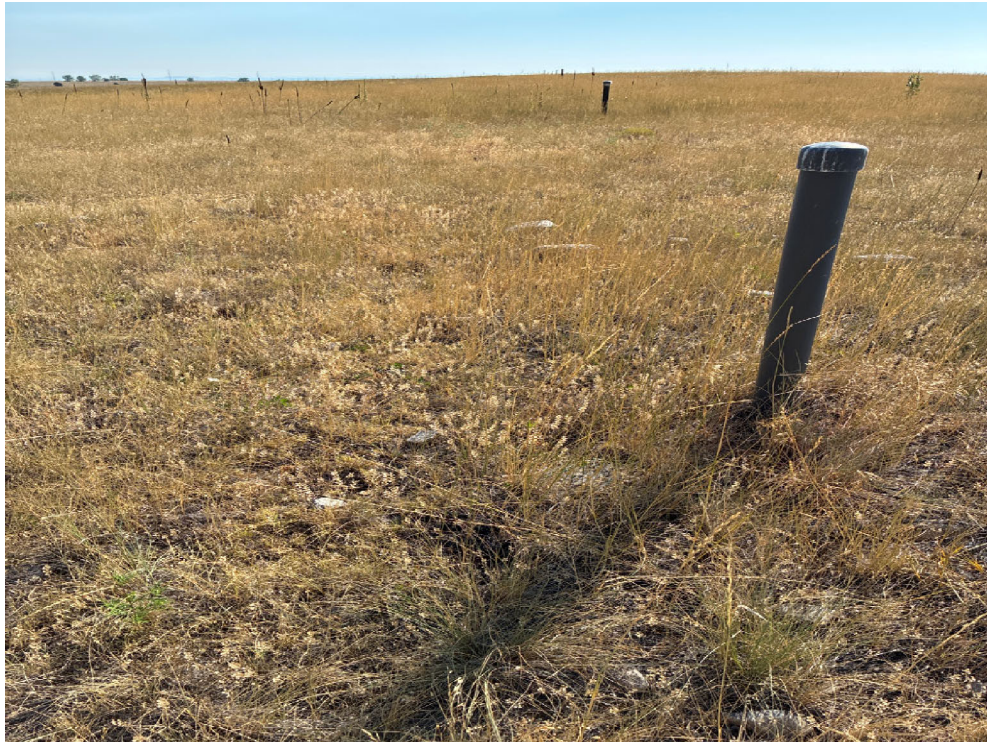
Figure 5. Looking East at Settlement Monuments and Barometric Gas Vents on the Present Landfill Cover, Which Were in Good Condition.
