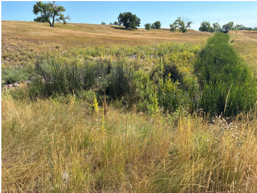
Figure 9. View Looking East at the SID, Which Receives Groundwater from the ESDD Outfall and an Interceptor Drain on the Eastern Hillside and Had a Flow Rate of Approximately 1–2 gpm
