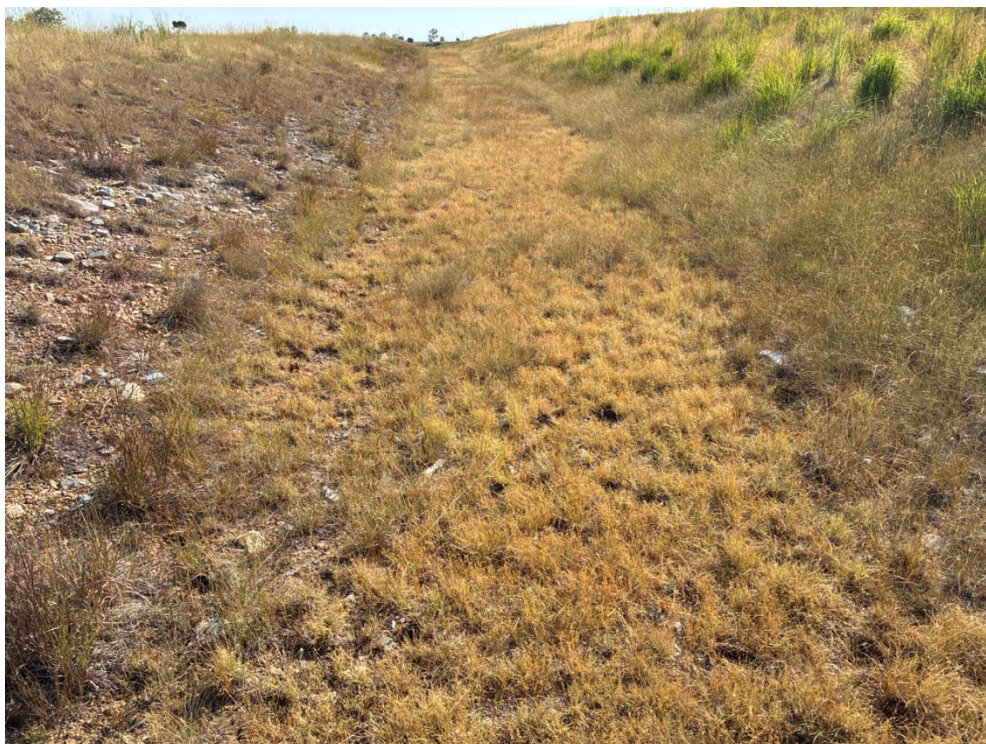
Figure 4. Looking Northeast at the Northern Vegetation-lined Perimeter Channel, Which Was in Good Condition.
