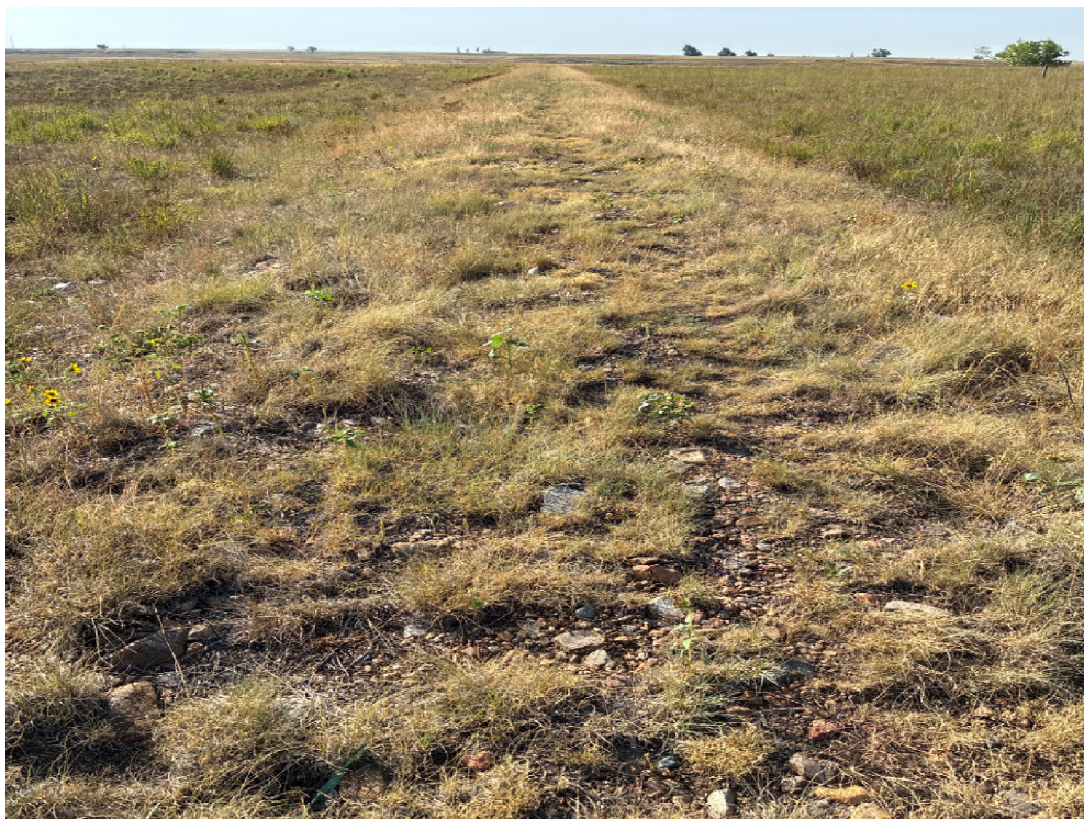
Figure 3. Looking South at a Diversion Berm that Runs Along the Eastern Pediment, Which Was in Good Condition.
