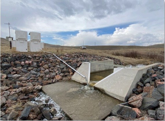
Walnut Creek Point of Compliance
