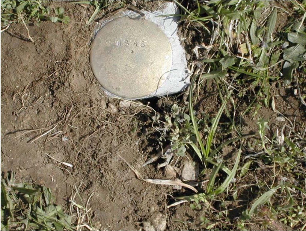
Photo 3: Repaired WS-46 Monument. Located on Army Property.
