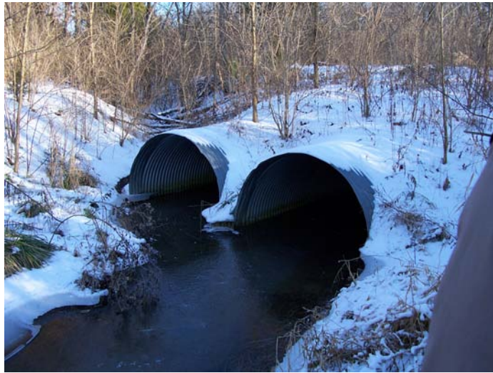
Photo 7. Highway D culverts.
