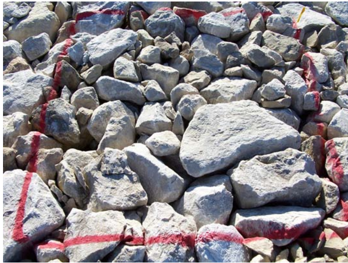
Photo 11. Cell cover rock test plot TP1; north edge of north facet (2006 Inspection).
