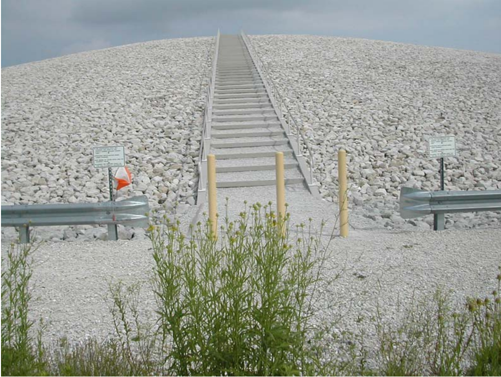
Photo 7: New signs posted at bottom of disposal cell at access stairway.
