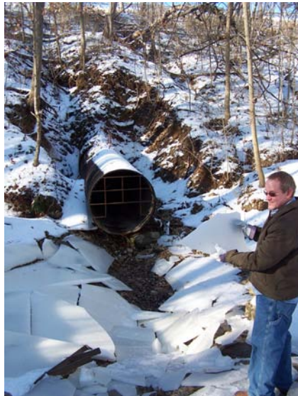
Photo 8. Highway 94 culvert outlet in the Southeast Drainage.
