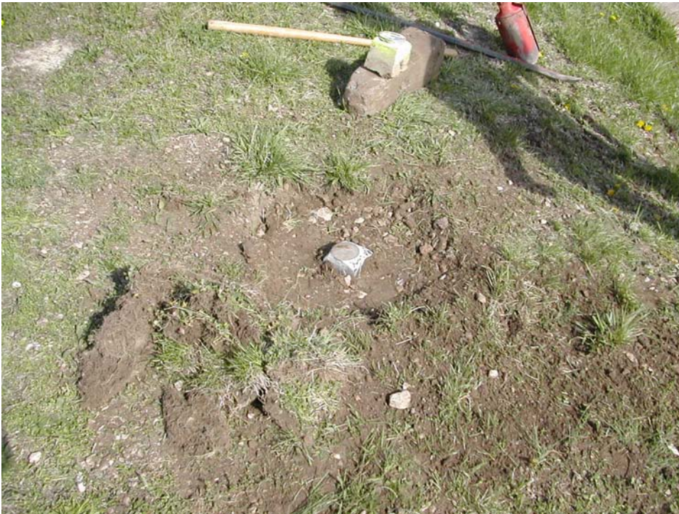
Photo 2: Monument WS-46 Repair. Located on Army Property.
