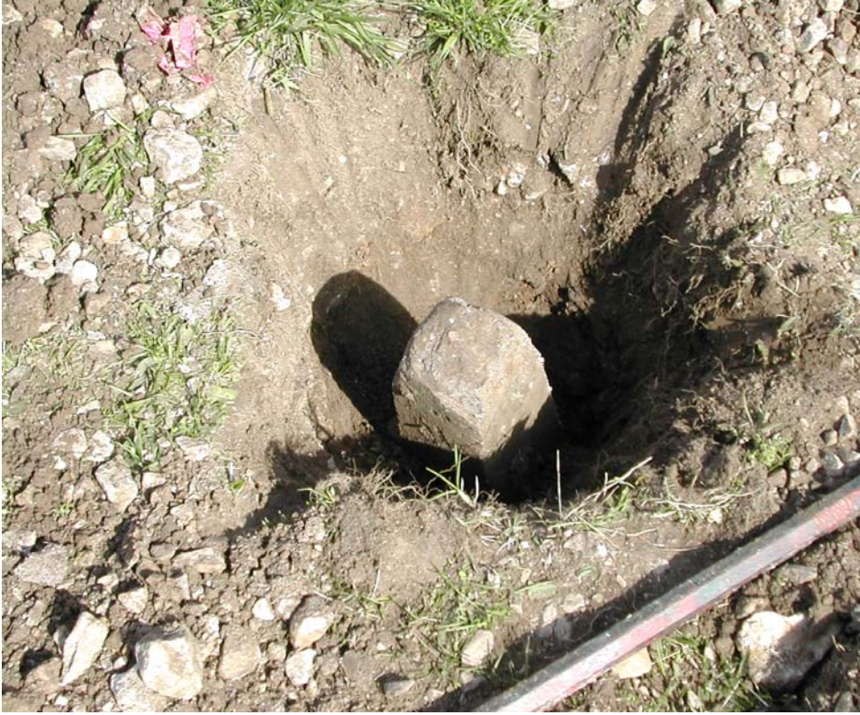
Photo 1: Monument WS-46 Repair. Located on Army Property.
