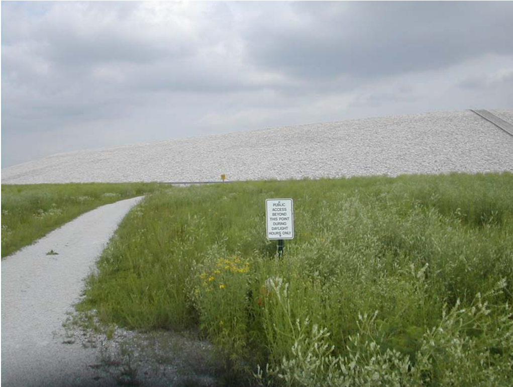
Photo 5: New sign posted at access road to disposal cell.
