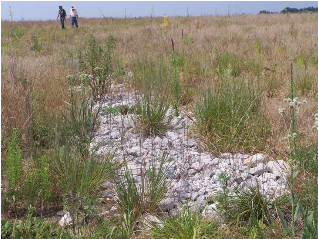
Photo 5: View upslope of repaired gully in Area #5; this repair is effectively controlling erosion.
