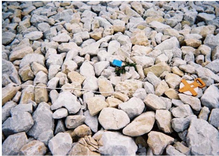
Photo 19. Cell cover rock test plot TP4; located on upper west side (2003 Inspection).
