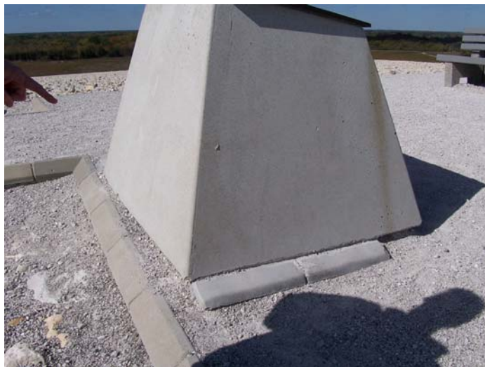
Photo 27. Repair of erosion under the monument on the disposal cell
