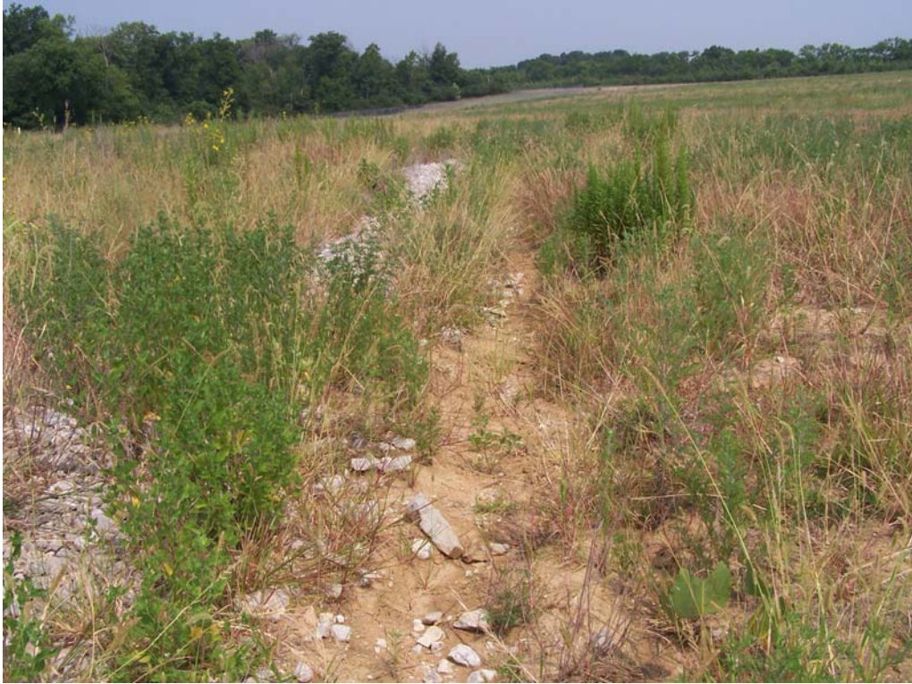
Photo 6: View downslope of repaired gully near Area #3 and newer rill forming to the right of the repair; note vegetation in bottom of rill.
