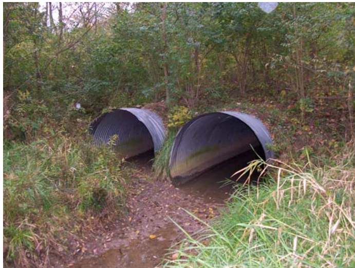
Photo 6. Highway D culverts.
