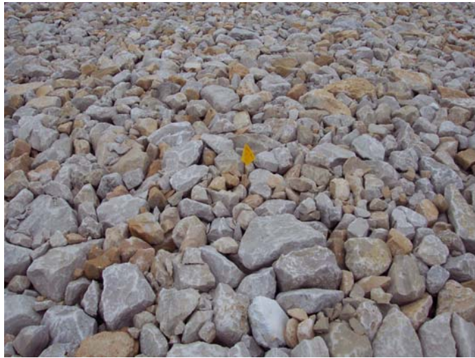
Photo 10. Cell cover rock test plot TP1; north edge north facet (2003 Inspection).
