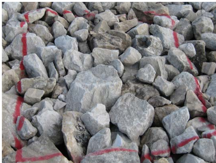
Photo 24. Cell cover rock test plot TP5; located on lower west side (2007 Inspection).
