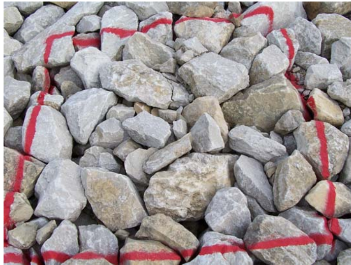
Photo 20. Cell cover rock test plot TP4; located on upper west side (2006 Inspection).
