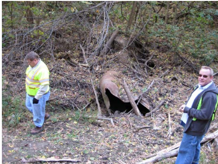
Photo 7. Highway 94 culvert inlet in the Southeast Drainage.
