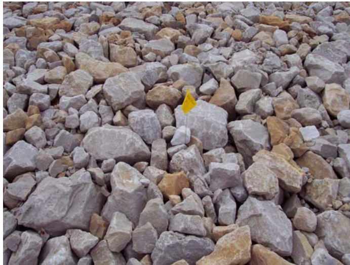
Photo 13. Cell cover rock test plot TP2; bottom of north side slope (2003 Inspection).
