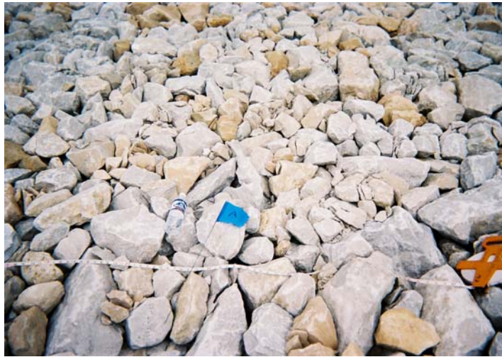
Photo 16. Cell cover rock test plot TP3; northeast ridgeline (2003 Inspection).
