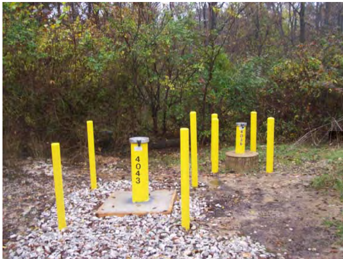
Photo 2. Monitoring well MW-4043 on the Army Property.
