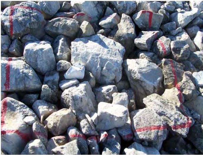
Photo 11. Cell cover rock test plot TP2; north edge north facet (2008 Inspection).
