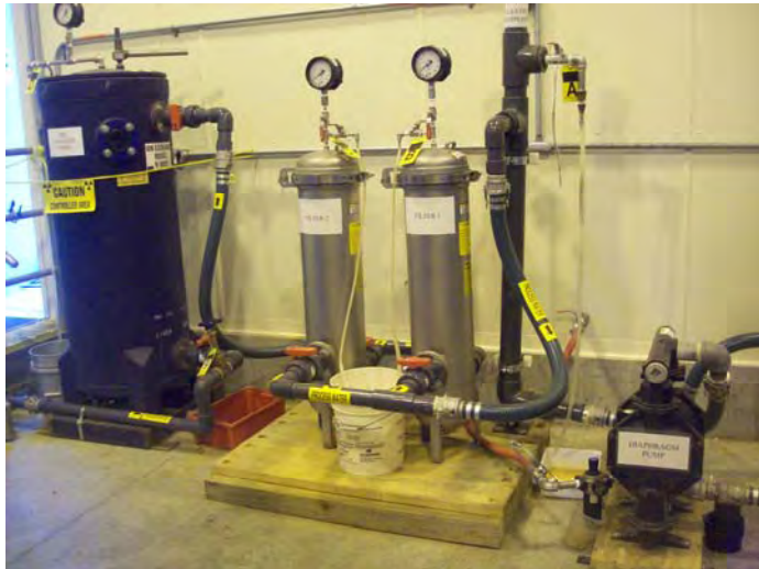
Photo 22. Inside LCRS Building.
