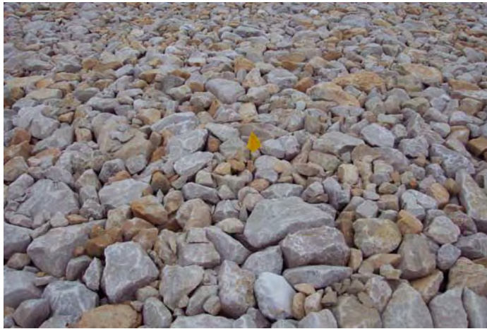
Photo 7. Cell cover rock test plot TP1; north edge north facet (2003 Inspection).
