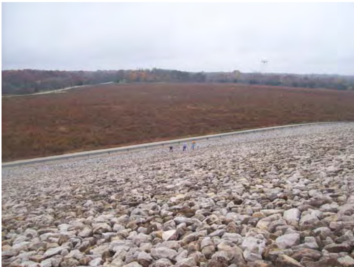
Photo 6. Disposal cell inspection looking south.
