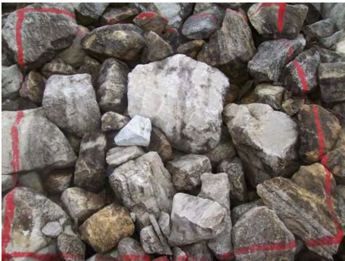
Photo 12. Cell cover rock test plot TP2; north edge north facet (2009 Inspection).
