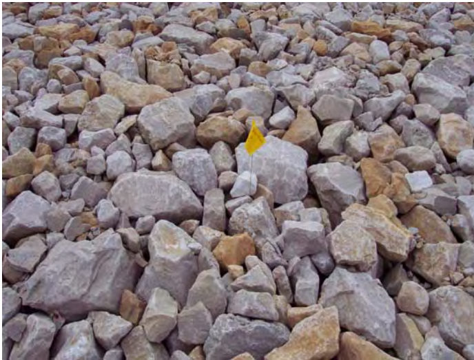
Photo 10. Cell cover rock test plot TP2; north edge north facet (2003 Inspection).
