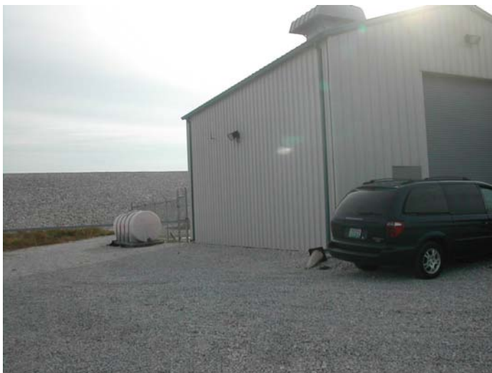
Photo 20. Outside Train 3 LCRS Building.
