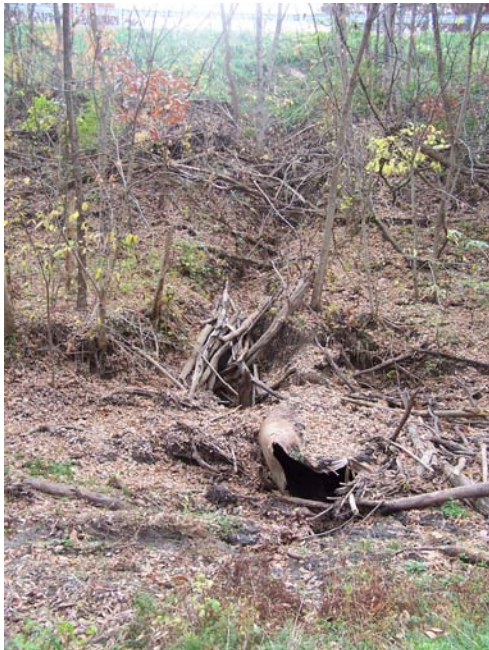
Photo 12. Highway 94 culvert inlet in the Southeast Drainage.
