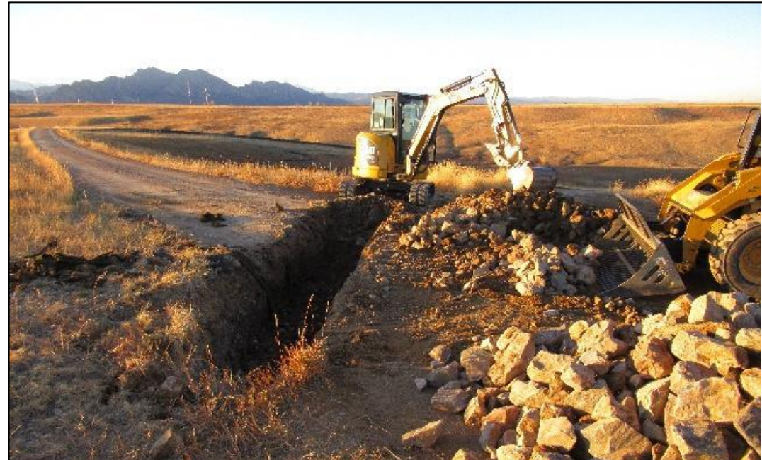
Rock crossing repair
