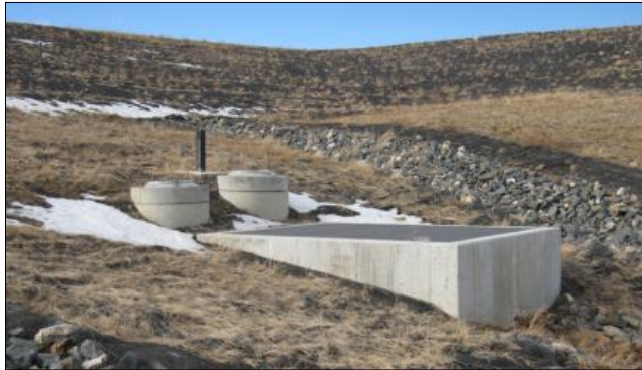
Present Landfill Treatment System (PLFTS)
