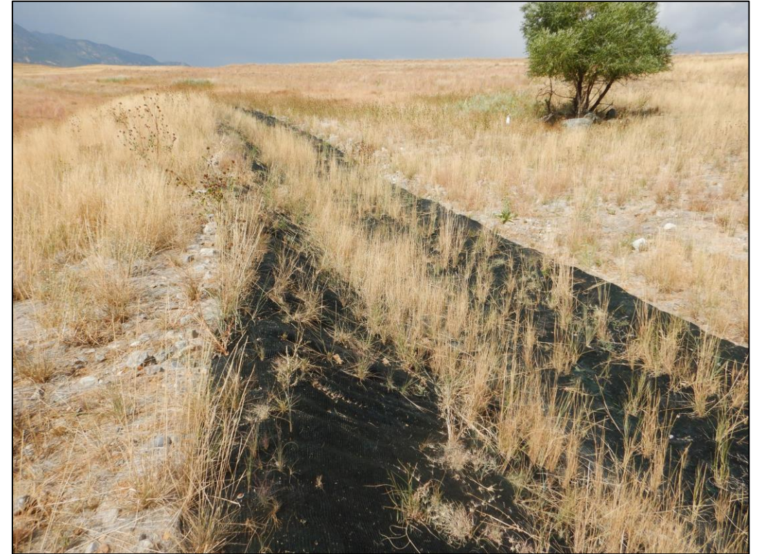
Berm Seven of the OLF with turf reinforcement mat
