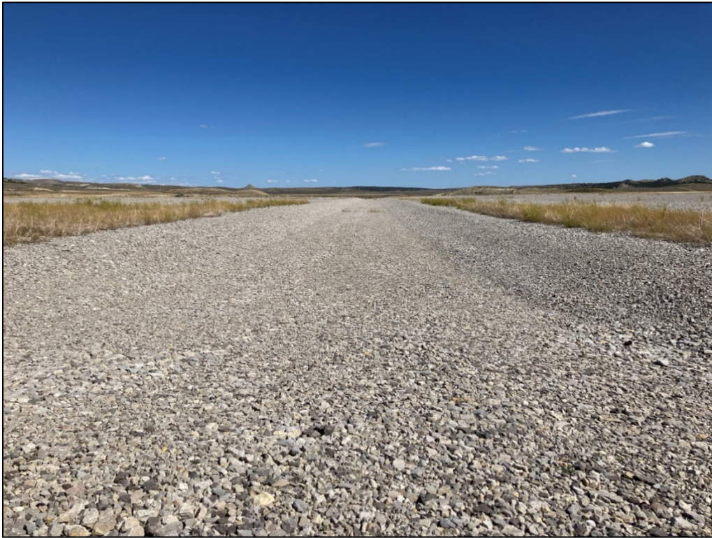
PL-10. Diversion Channel No. 1
