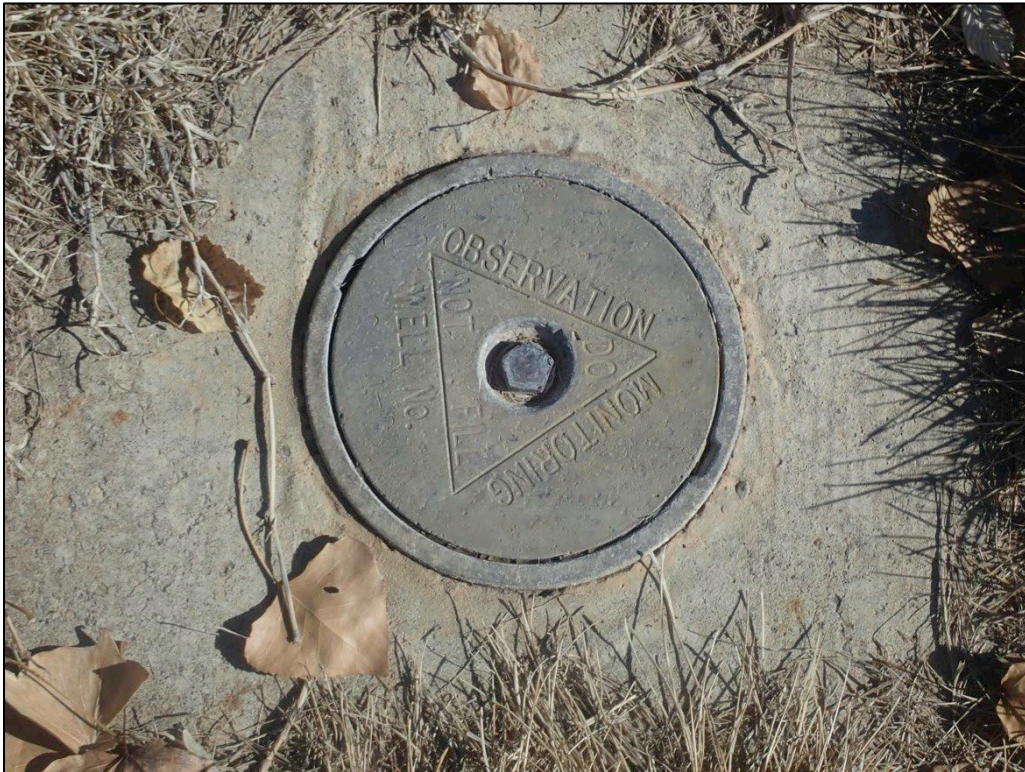
PL-2. Monitoring Well GJ01-02
