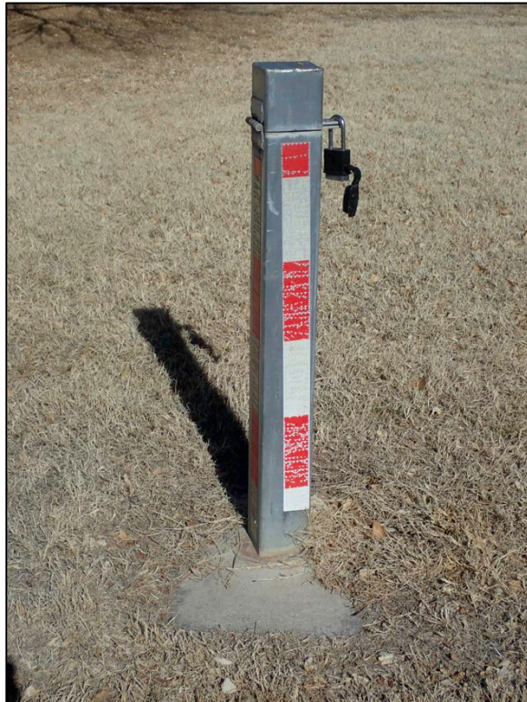
PL-4. Monitoring Well GJ01-01
