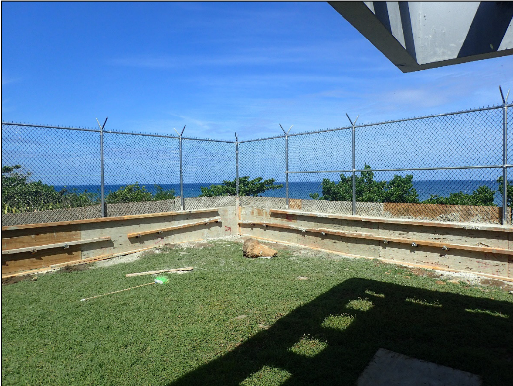
PL-7. New Perimeter Wall and Fence
