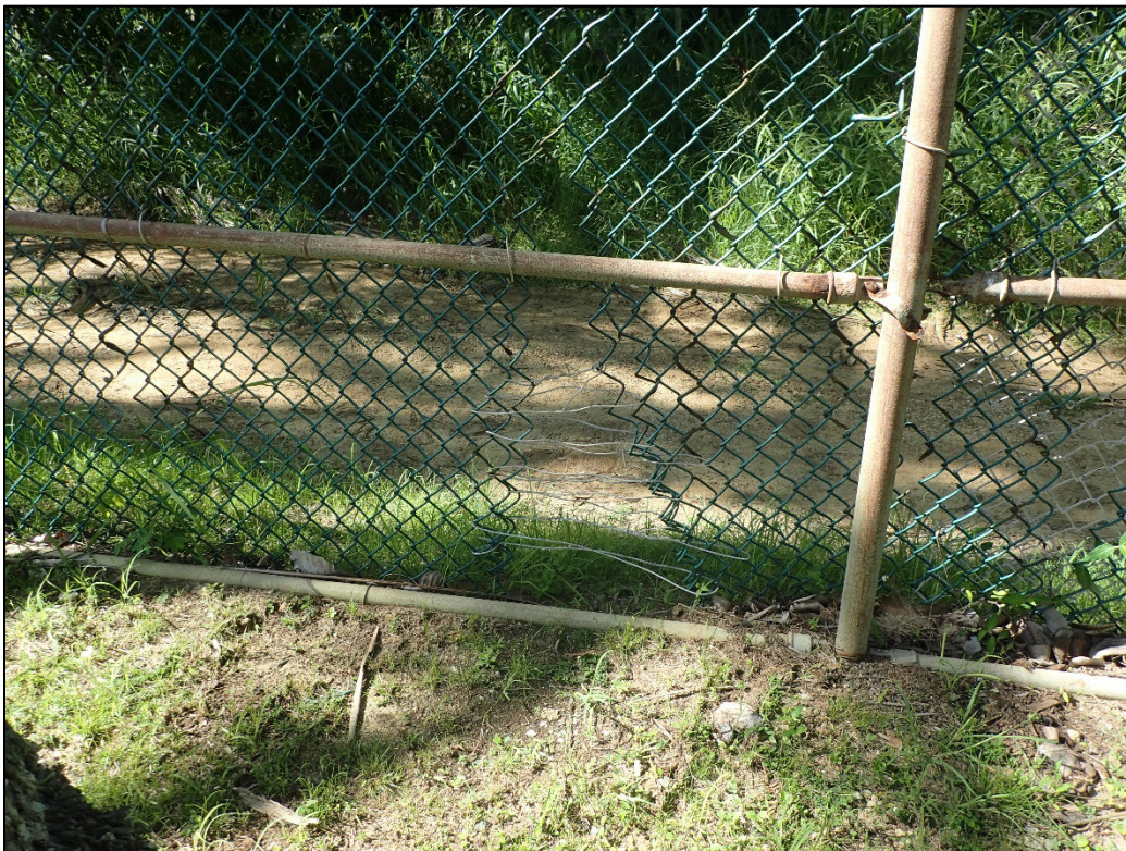
PL-5. Perimeter Fence Repair
