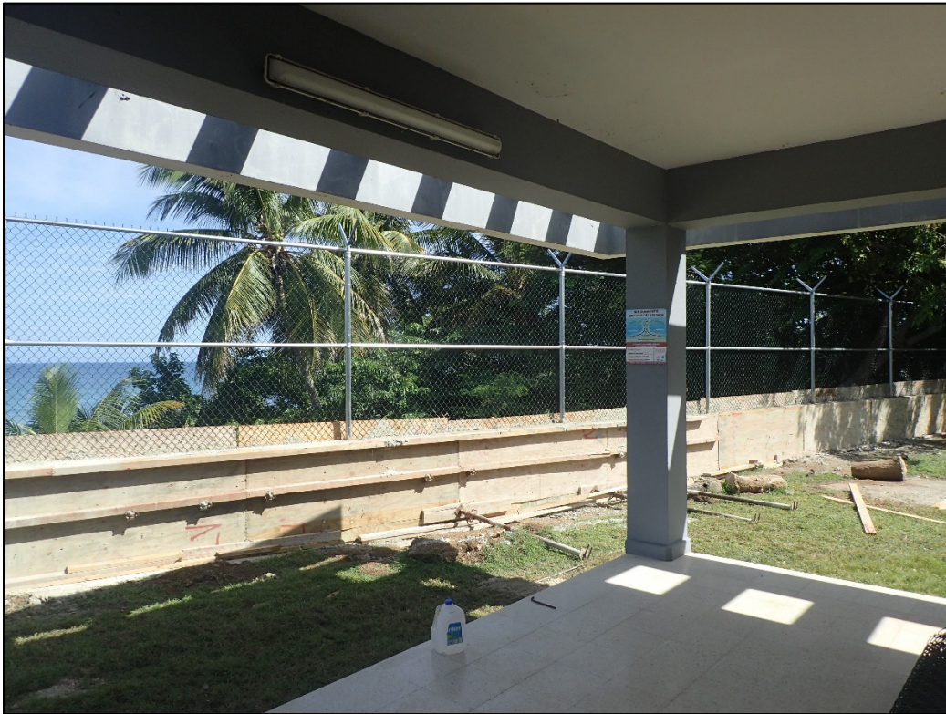
PL-8. New Perimeter Wall and Fence
