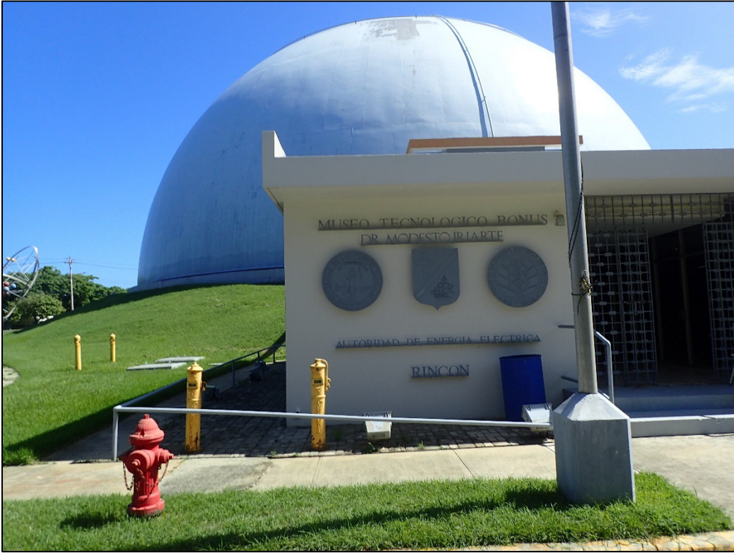
PL-2. Containment Dome
