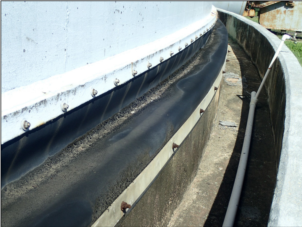
PL-3. Seal Along Base of Dome
