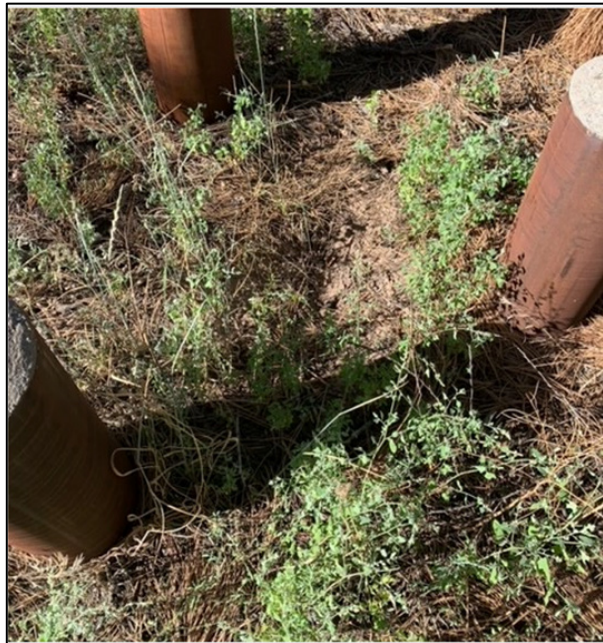
Photo 4. Location of Missing Site Marker #1/Monument A (Center of Bollards)
