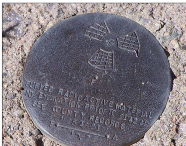
Photo 5. Example of Missing Site Marker
