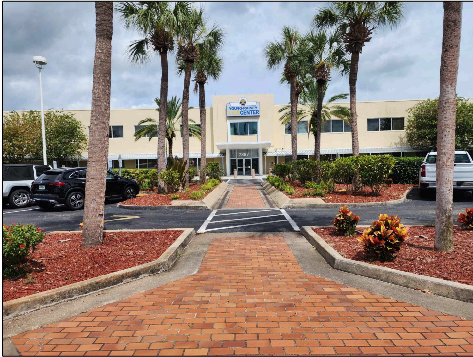
Photo 3. Building 100, Looking North
