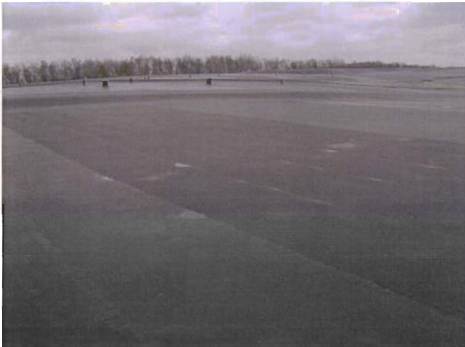
Photo 10: Liner Overview from South East Quadrant Looking North West
