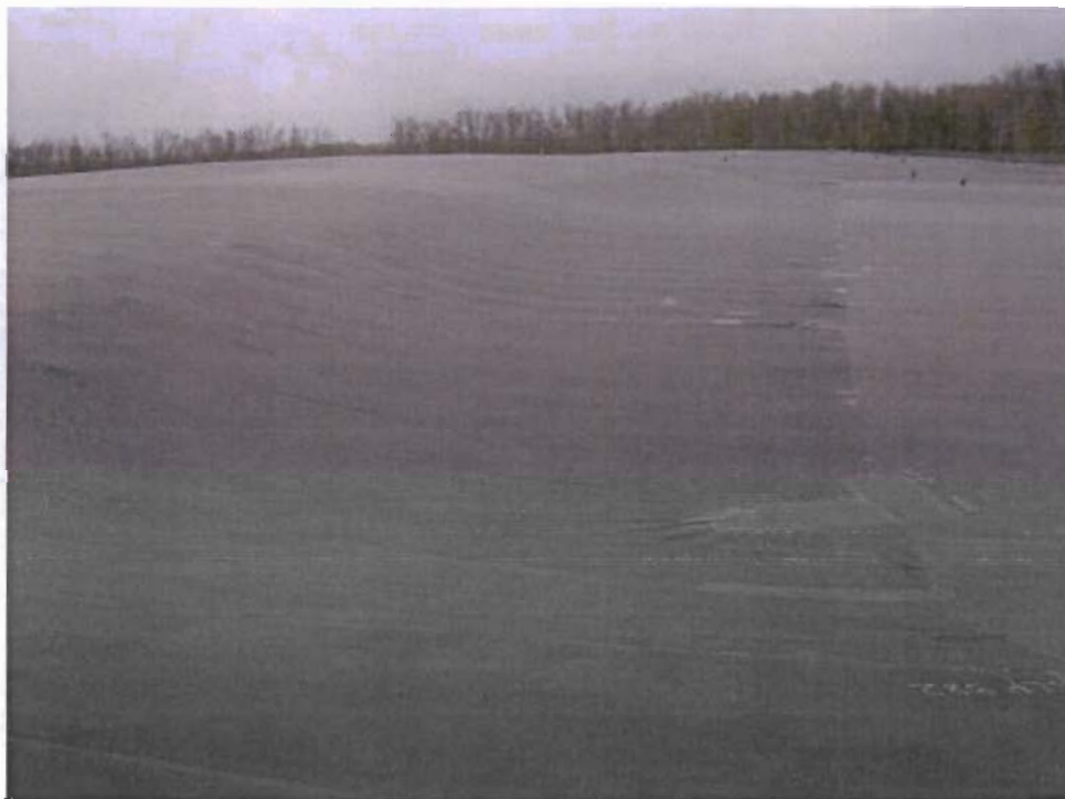
Photo2: North West Quadrant Looking South – Typical Bunker Slopes
