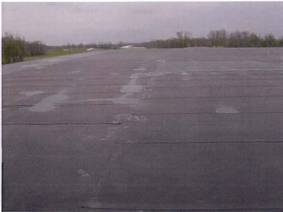
Photo1: North West Quadrant Liner Overview – Looking North
