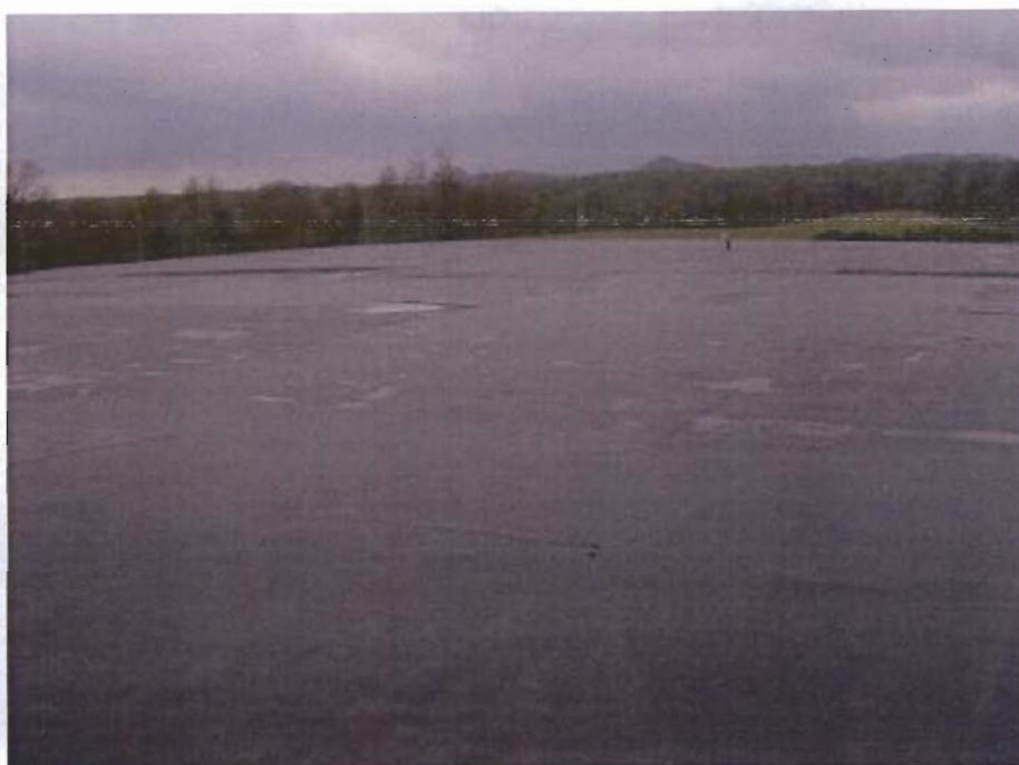
Photo 7: Liner Overview from Northern Area Looking South
