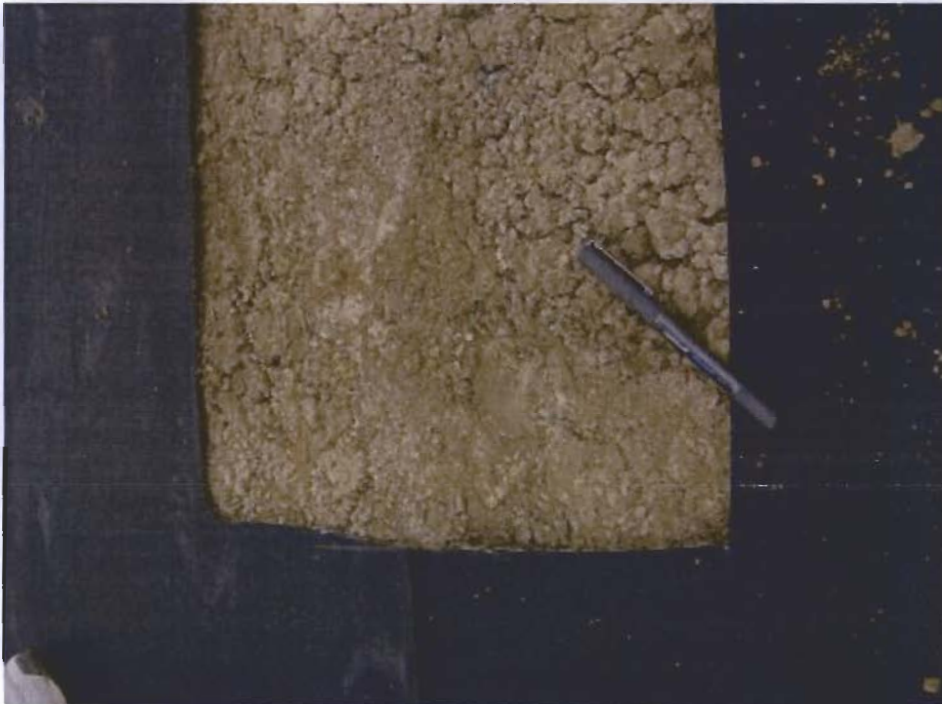
Photo 12: Desiccated Soil Subgrade at LE-1
