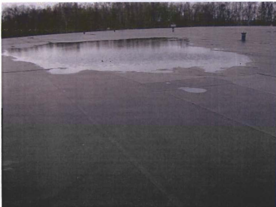
Photo 5: Ponded Water in South Central Area
