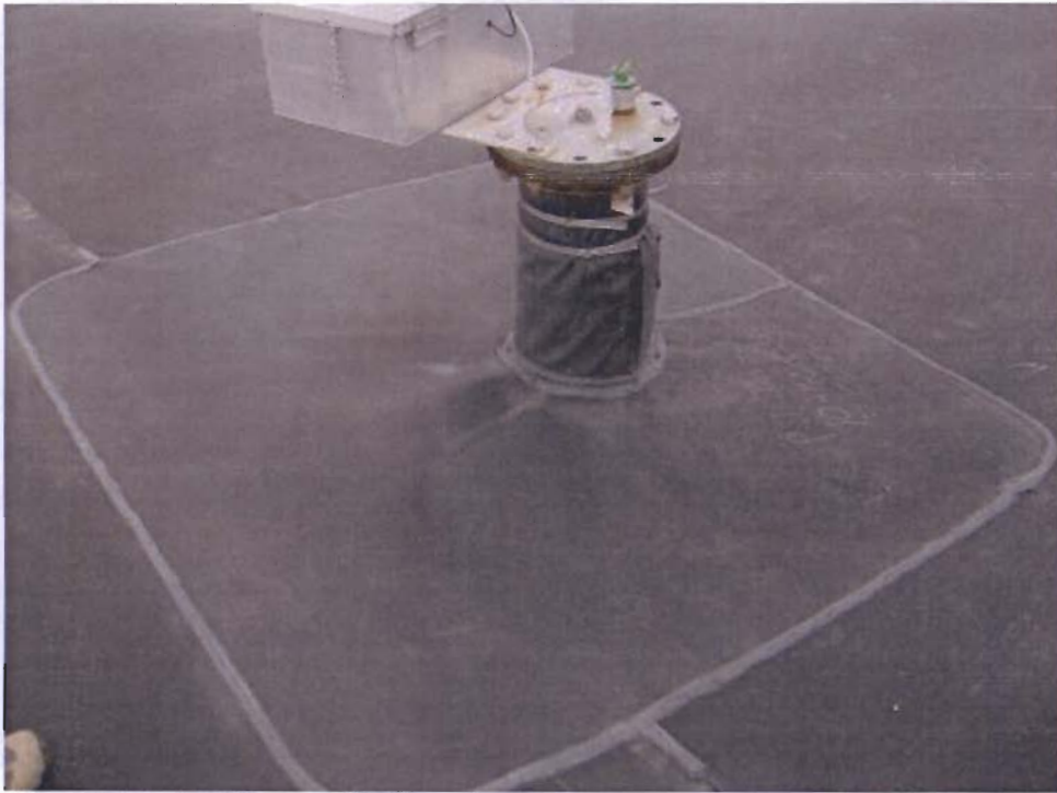
Photo 3: Typical Sump with Liner Boot
