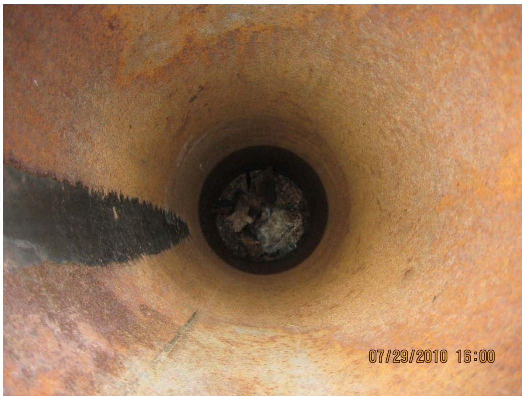
Photograph 24 – View inside Test Hole X1 casing.
