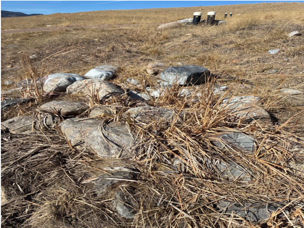
Figure 9. View Looking West-Northwest at the ESSD, Which Had a Flow Rate of Less Than 1 gpm
