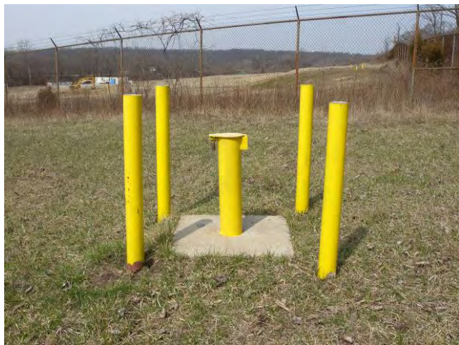
Figure 27. Parcel IC Well 0445, Locked, Labeled, and in Good Repair
