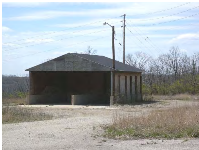
Figure 20. Phase IB Empty Salt Storage Shed
