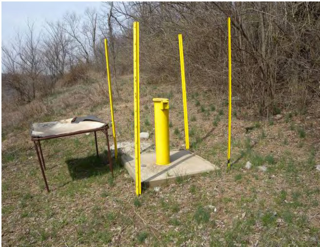
Figure 23. Parcel IB Well 0443, Locked, Labeled, and in Good Repair
