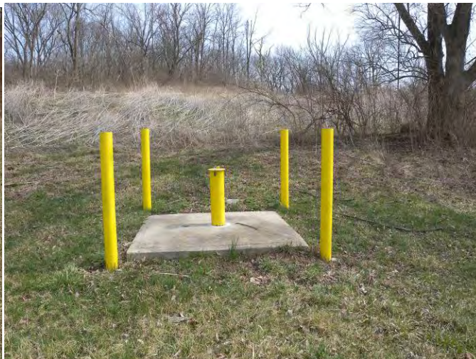
Figure 28. Parcel IC Well 0400, Locked, Labeled, and in Good Repair
