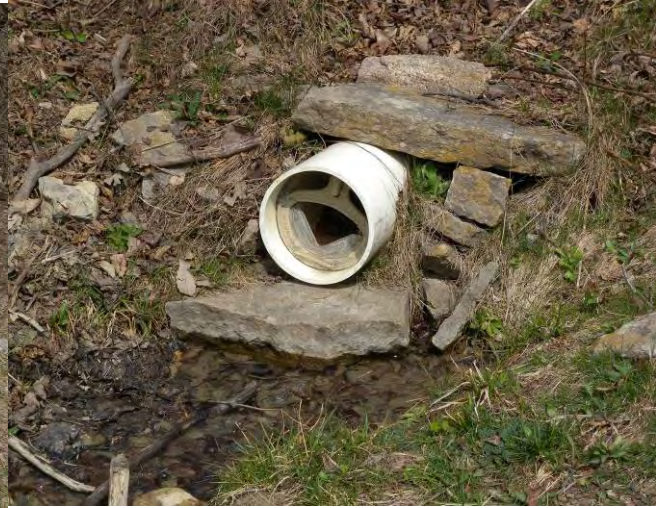
Figure 24. Parcel IB Groundwater Seep 0617
