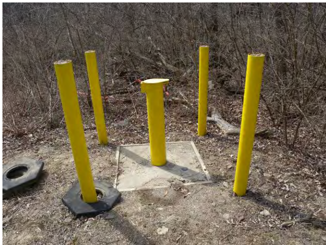
Figure 13. Parcel 4 Well 0444, Locked and in Good Repair
