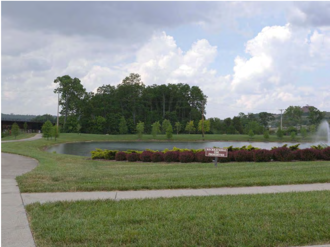
Figure 12. Parcel 4 MMCIC Retention Pond with New Signage. Bike Path at Left of Photo.
