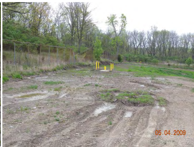
Figure 33. Parcel 9 MNA Well 0353 Showing Drainage Problem North of Well
