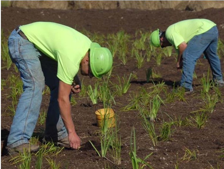
Fig. 2. Field personnel install herbaceous plugs into the subsurface flow wetland.
