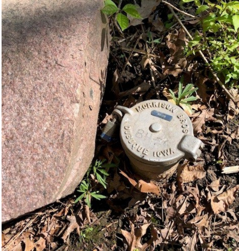
P07 - Monitoring Well BH26 at Plot M
