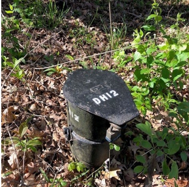
P14 – Monitoring Well DH12 at Red Gate Woods
