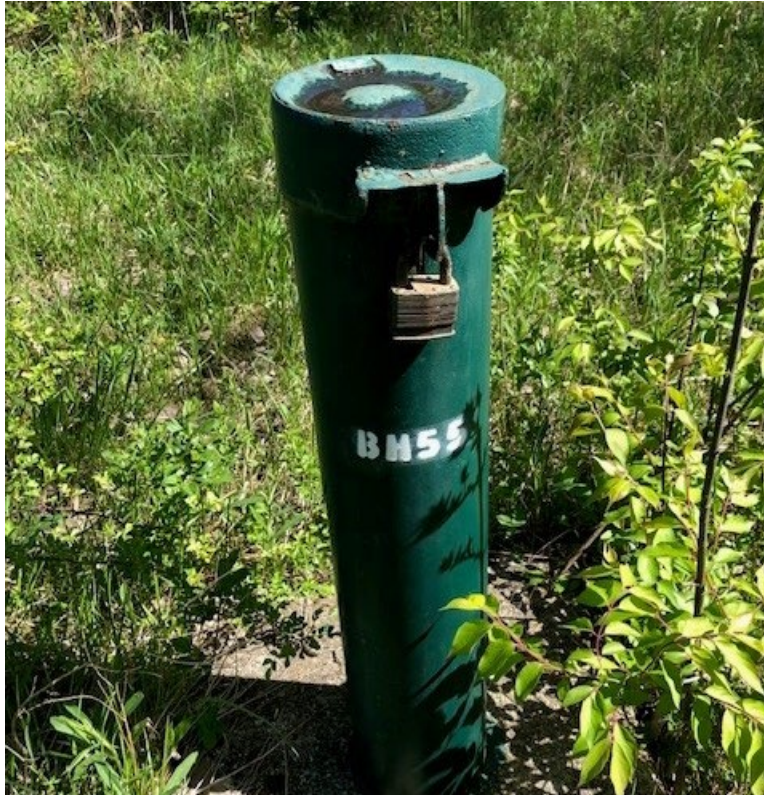
P9 – Monitoring Well BH55 at Site A
