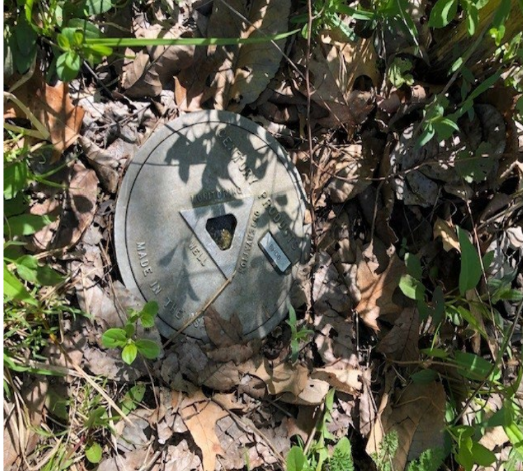
P03 – Monitoring Well BH06 at Plot M
